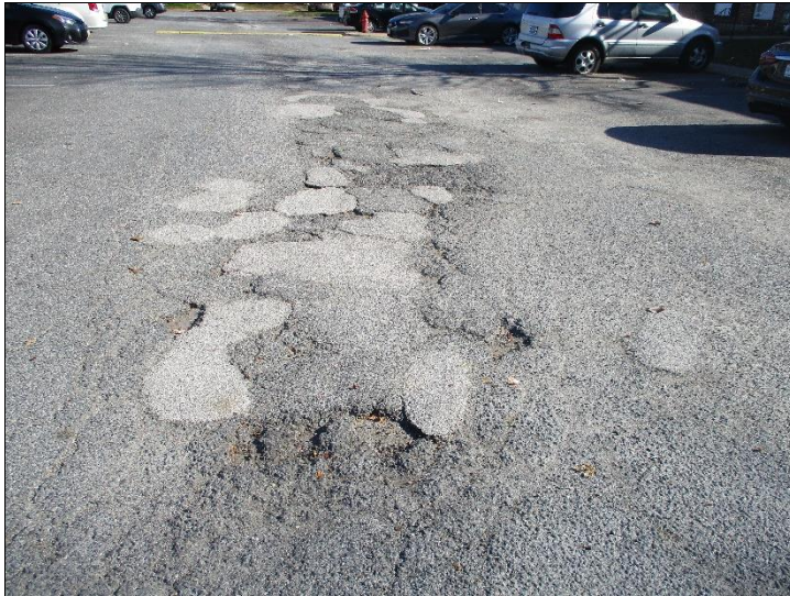
Photo #1: The asphalt has failed and should be considered for a mill and overlay.
