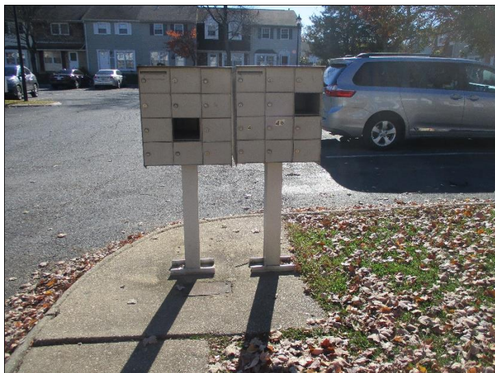
Photo #7: The mailbox pedestals have reached the end of their useful life and should be replaced.
