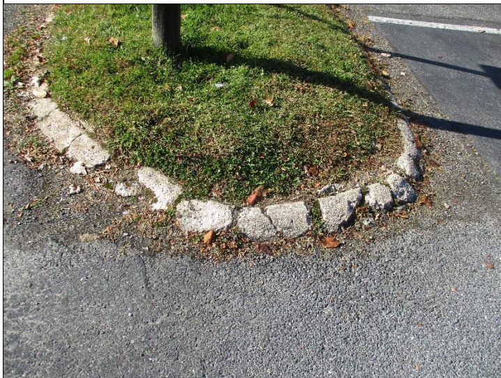
Photo #5: Damaged curbs were also noted. We recommend replacing the damaged curbs.
