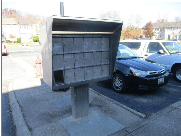
Photo #8: The mailbox pedestals have reached the end of their useful life and should be replaced.
