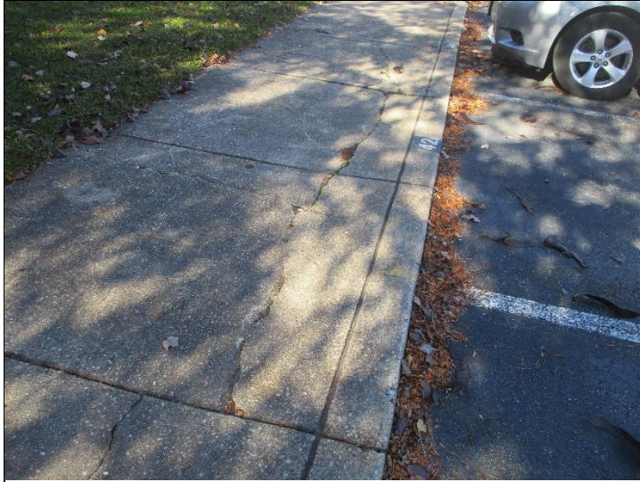
Photo #4: Several cracked and damaged concrete walks were noted.
