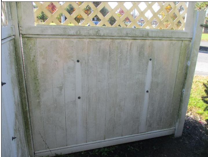
Photo #11: Areas of the PVC sign fencing was soiled during our review. Consideration should be given to power washing the fence for aesthetic purposes.
