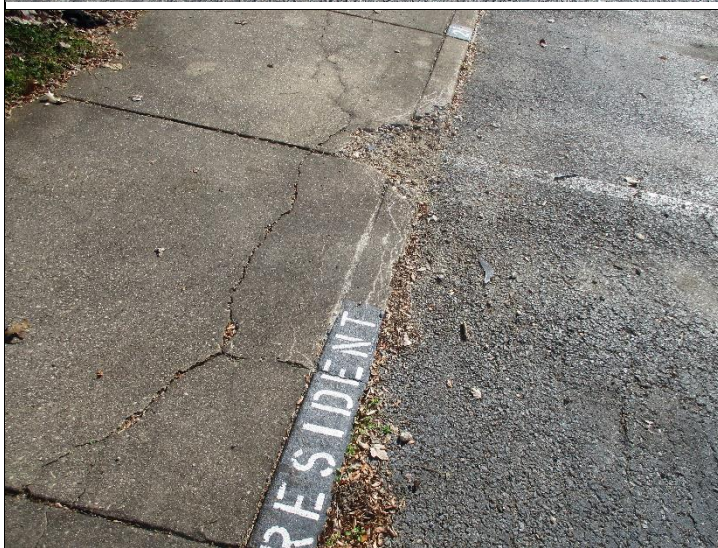
Photo #6: Damaged curbs were also noted. We recommend replacing the damaged curbs.
