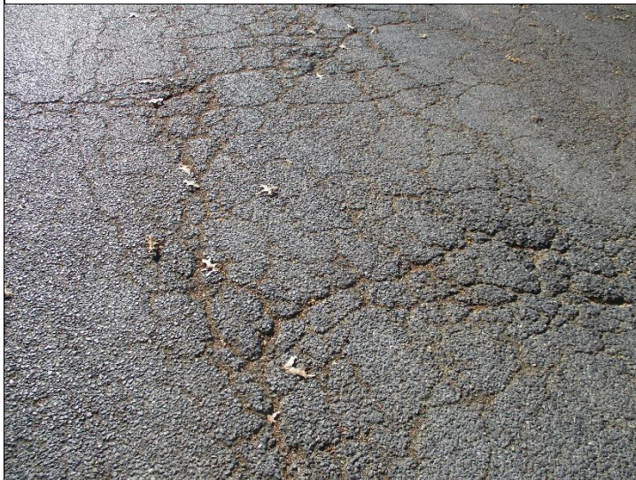
Photo #2: Areas with concentrated damage should be removed at full depth to make necessary repairs to the subbase before new asphalt is laid.
