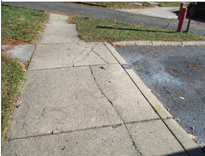
Photo #3: Several cracked and damaged concrete walks were noted.
