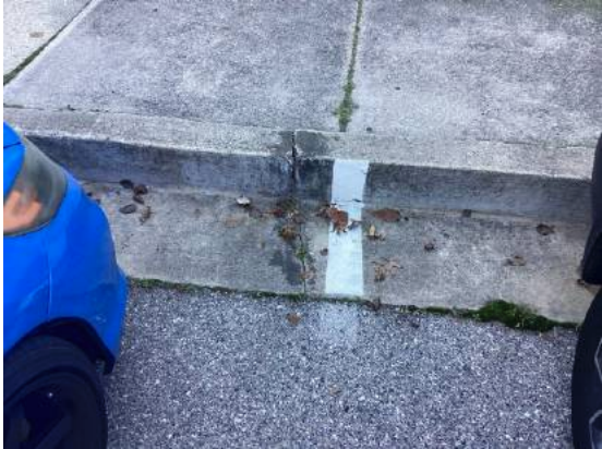
Concrete curb and gutter crack
