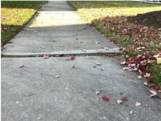
Sidewalk trip hazard
