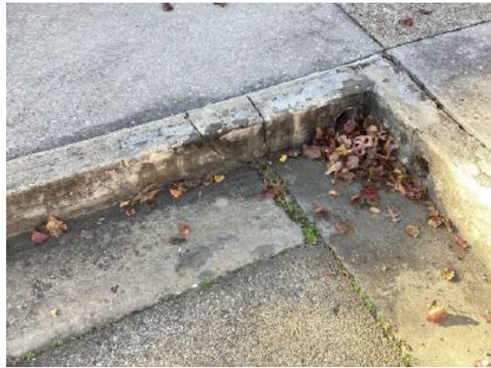
Concrete curb and gutter cracks
