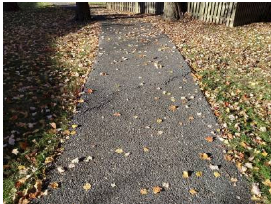
Walking path cracks
