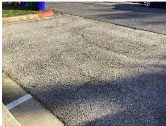
Pavement cracks
