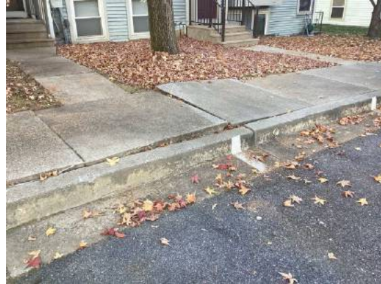
Sidewalk heave likely due to tree roots
