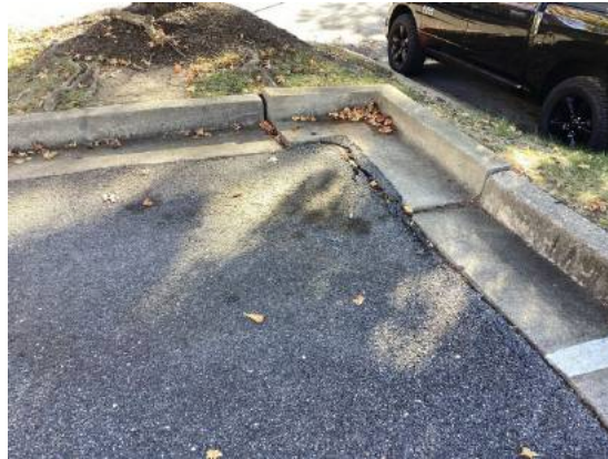
Pavement heave likely due to tree roots
