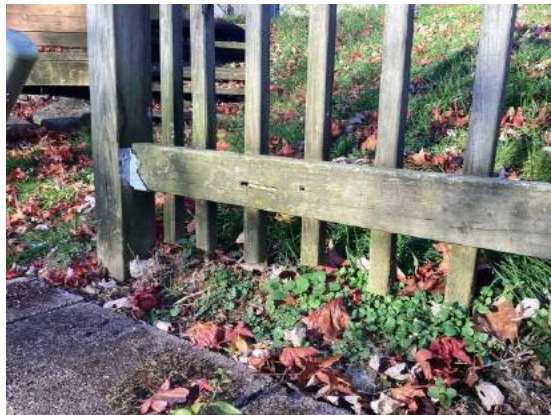
Wood rail deterioration
