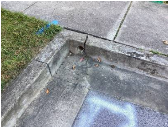
Concrete curb and gutter crack
