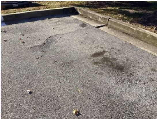
Pavement cracks and vehicular stains
