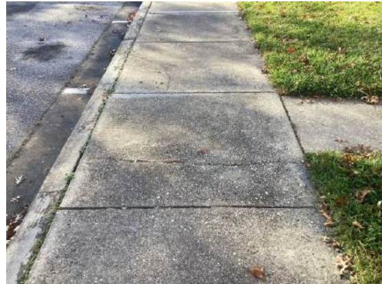
Sidewalk cracks
