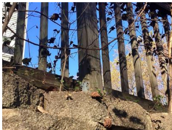
Wood post deterioration
