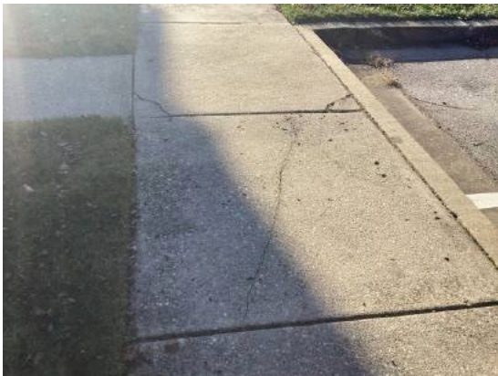
Sidewalk cracks
