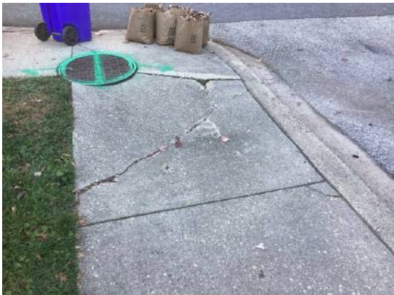
Sidewalk cracks
