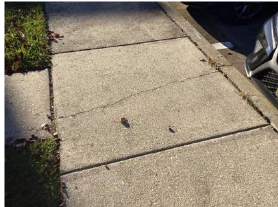
Sidewalk crack
