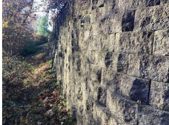
Masonry retaining wall
