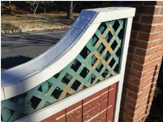
Sign finish deterioration
