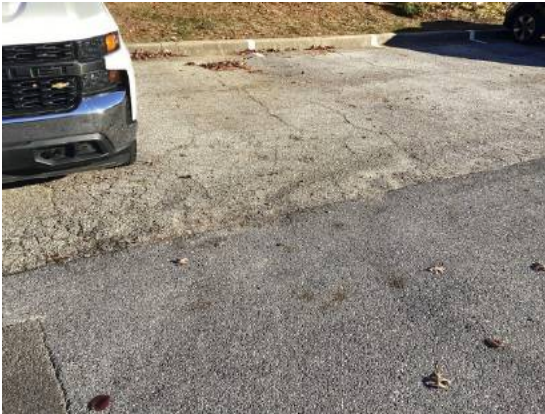
Pavement cracks
