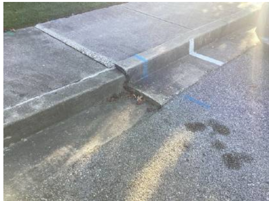
Concrete curb and gutter settlement
