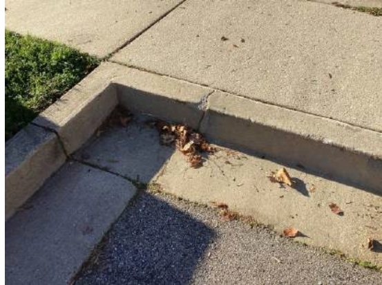
Concrete curb and gutter crack
