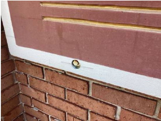
Sign deterioration and fastener rust
