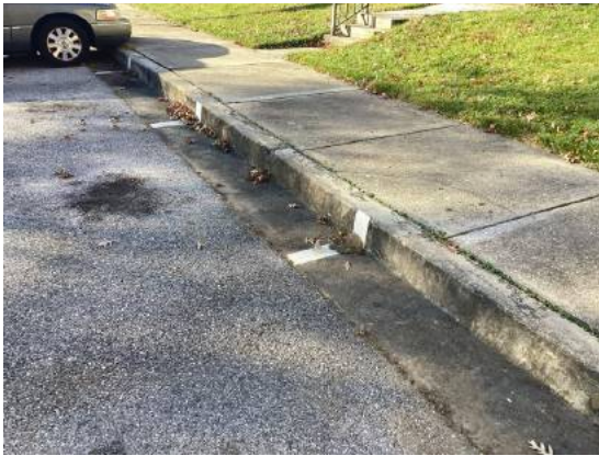
Concrete curb and gutter
