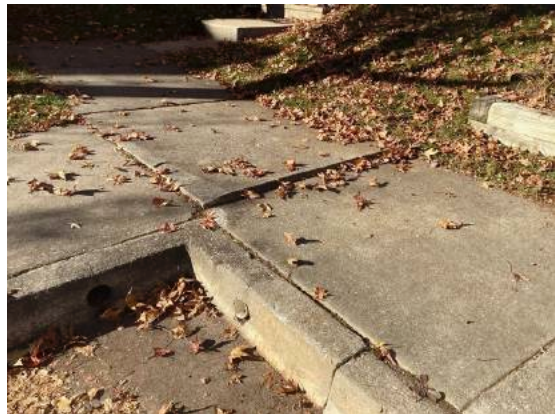
Sidewalk trip hazard
