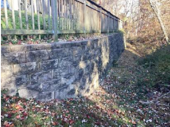
Masonry retaining wall
