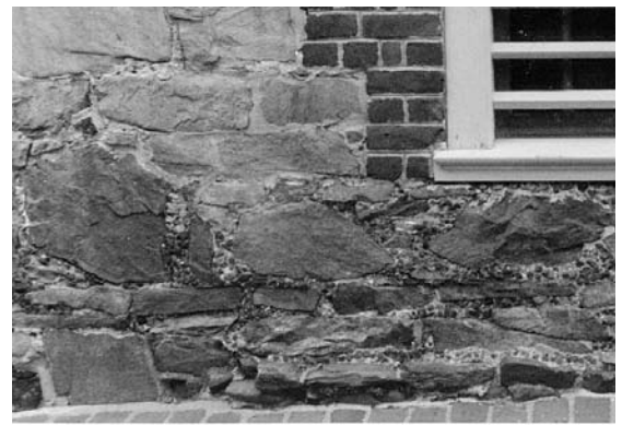
Figure 18 (above). Detail of galleting, William Paca House.
