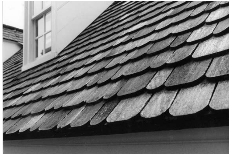
Figure 81. Detail of sawn shingle roofing, west dependency of the William Paca House.
