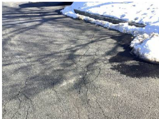
Cracks at the original pavement
