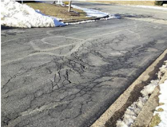
Cracks and previous repairs at the original pavement
