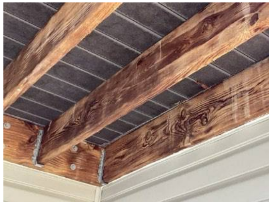
Wood deterioration
