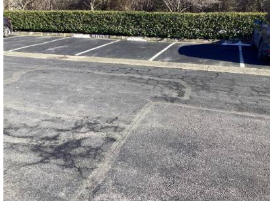
Cracks and patches at the original pavement
