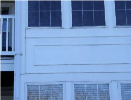
AZEK panel; we note weathered finish
