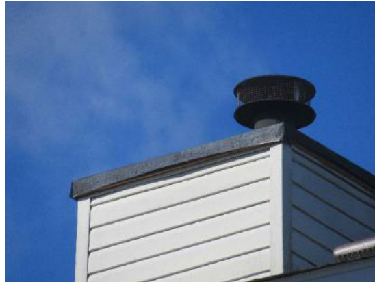
Warped chimney cap
