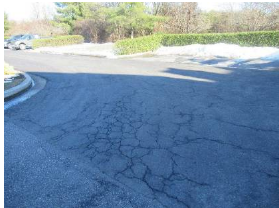
Cracks at the original pavement
