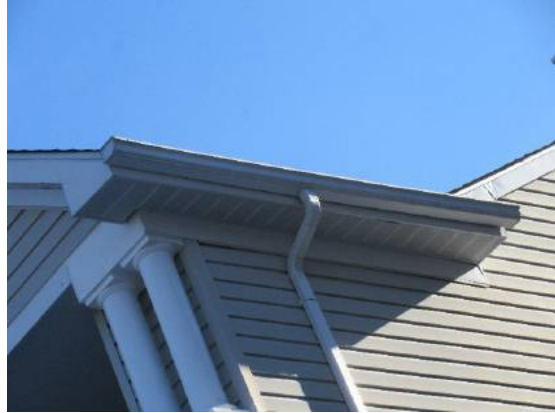
Gutters and downspouts
