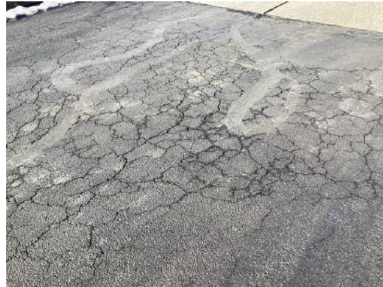
Alligator cracks at the original pavement
