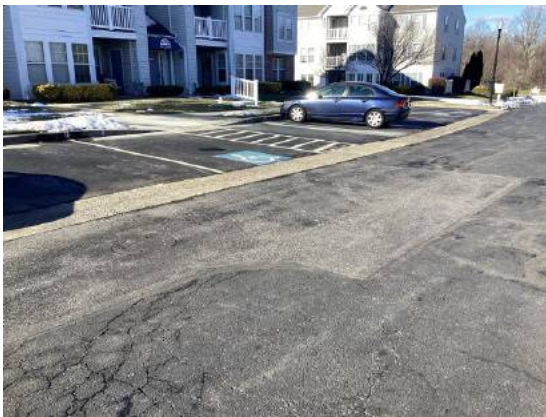
Cracks and patches at the original pavement
