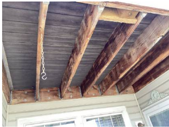
Balcony structure detail – Note previous partial replacements
