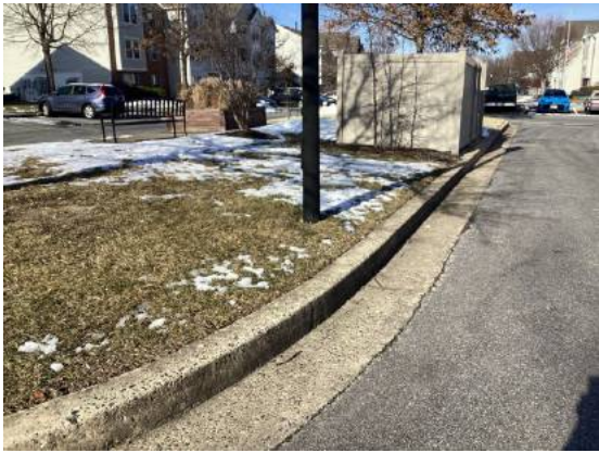
Concrete curb and gutter
