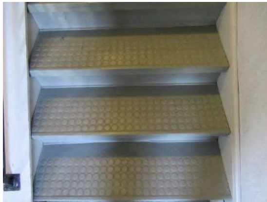
Rubber stair treads coverings
