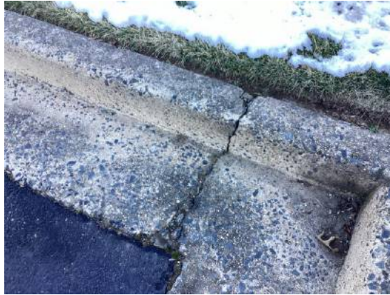
Concrete cracks
