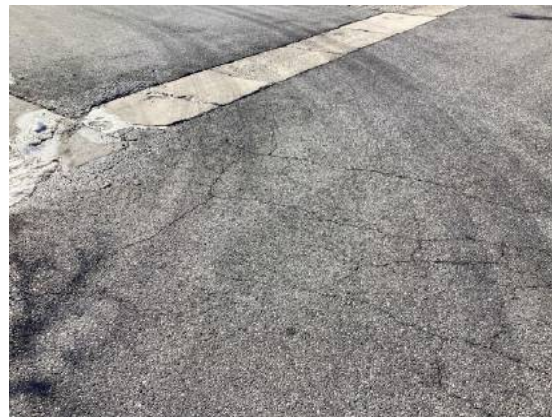
Cracks at the original pavement
