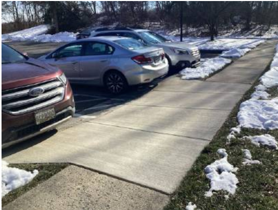
Concrete sidewalk - note partial replacements
