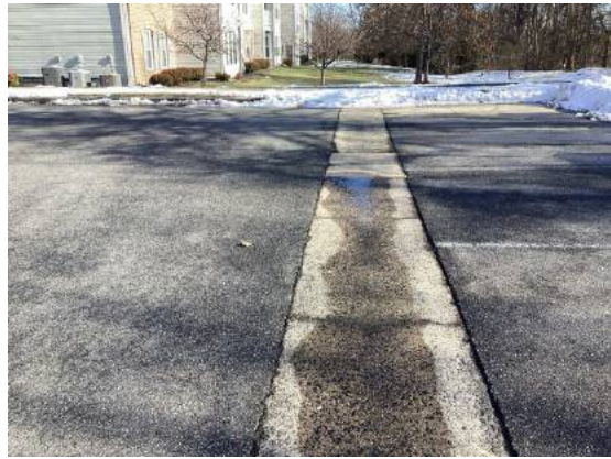
Concrete gutter
