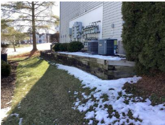
Timber retaining wall
