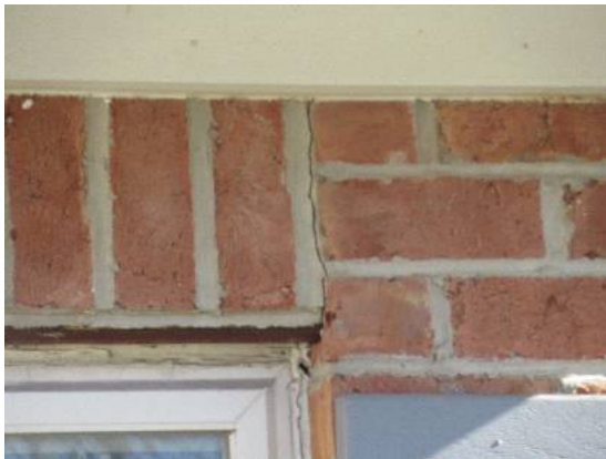
Cracks and lintel rust
