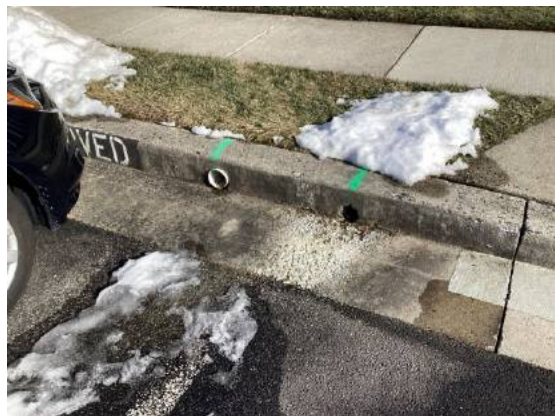
Concrete spalls and deterioration
