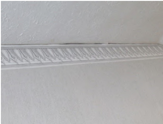
Stains and paint finish deterioration
