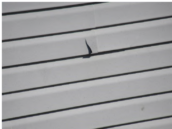
Damaged siding
