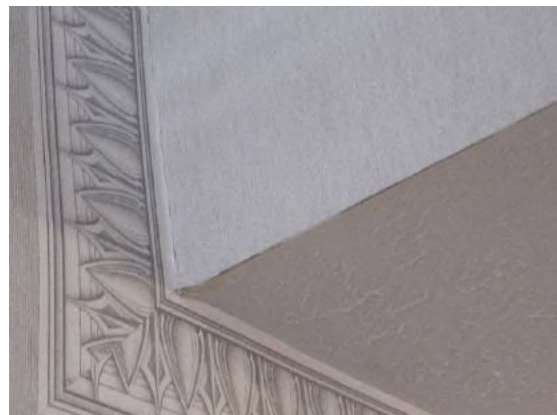
Paint finish deterioration
