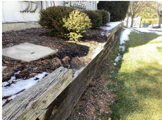
Wall excessive lean and missing timber sections
