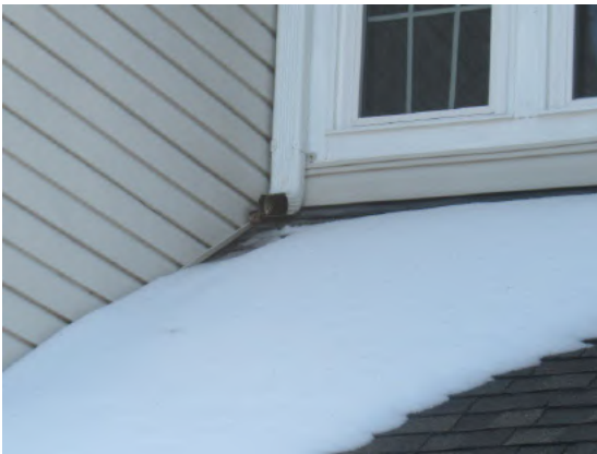
Downspouts discharge onto lower roofs
