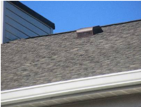
Shingle lift and sheathing deflection
