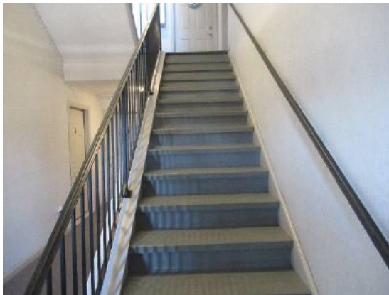
Rubber stair treads coverings
