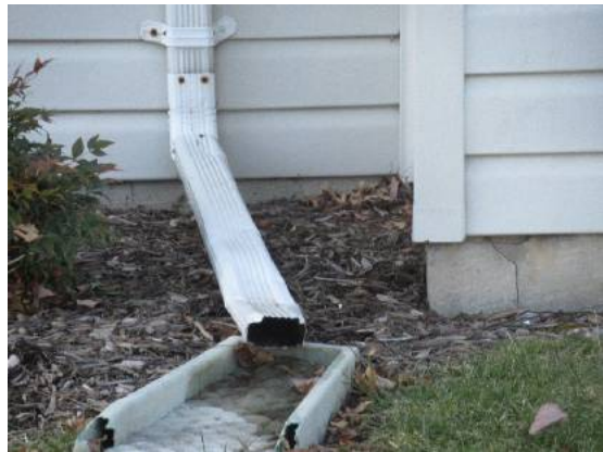
Dented downspout extension and rusted fastener
