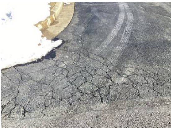
Alligator cracks at the original pavement
