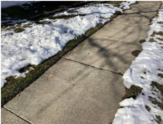
Sidewalk trip hazard
