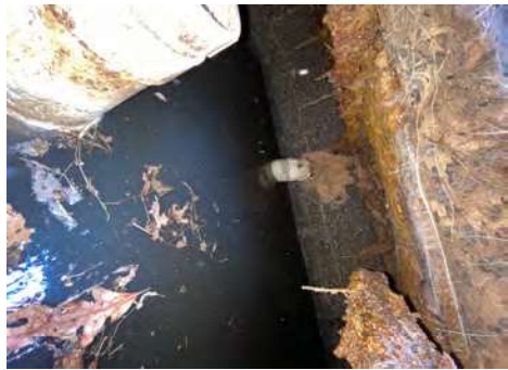
Inside of Cinder Block Tank
