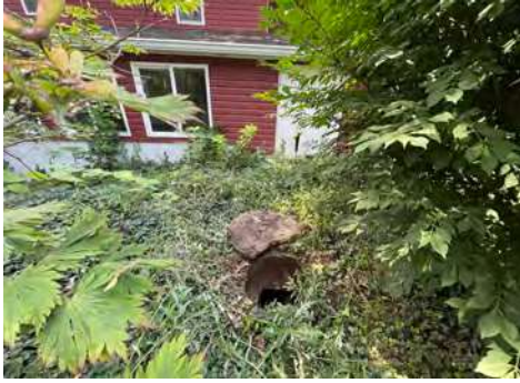
Cinder Block Tank Location
