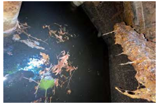
Inside of Cinder Block Tank
