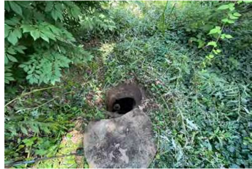
Cinder Block Tank Access
