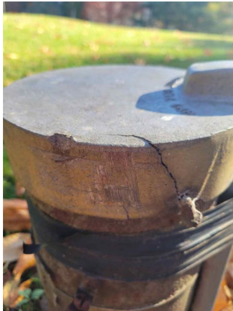
Cracked cap
