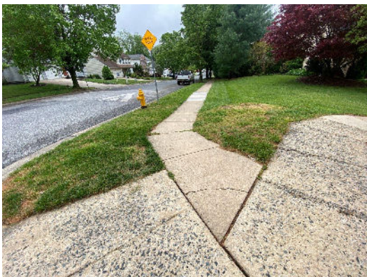
Concrete sidewalks - Gairloch Place & Redfield Road
