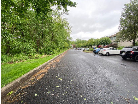
Recently repaved section of Kildonan Court
