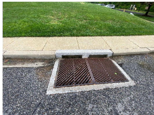
Typical storm drain, curb, and sidewalk - Kildonan Court
