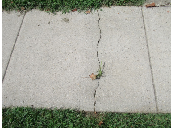
Sidewalk crack
