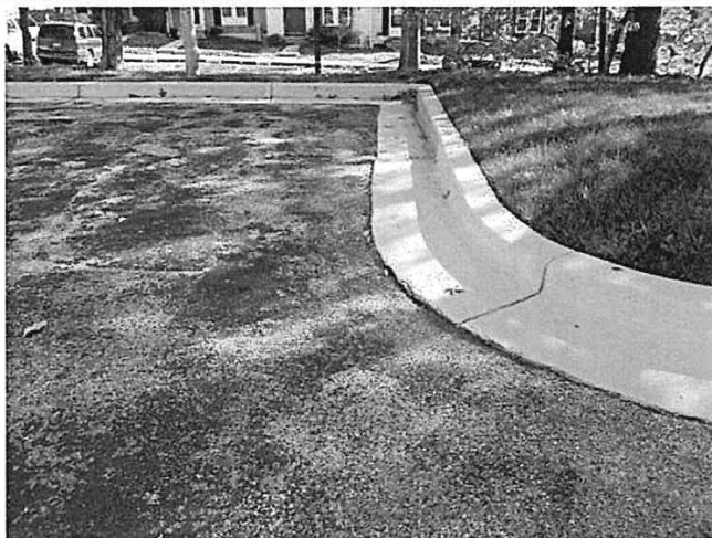
Abraded seal coat at Chipwood Court
