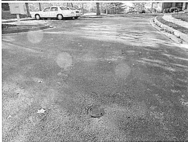
Asphalt pavement at Steepridge Drive
