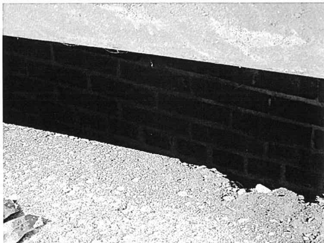
Brick walls within catch basin
