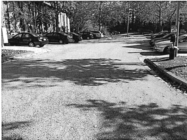
Diggers Lane pavement
