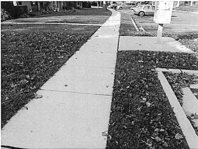
Typical concrete sidewalk
