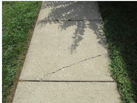
Sidewalk crack
