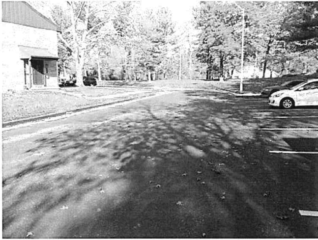
Asphalt pavement at Hunt Hill Drive
