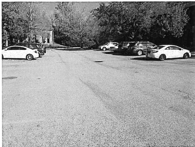
Diggers Lane pavement
