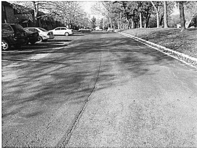
Asphalt pavement at Hunt Hill Drive
