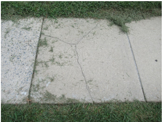
Sidewalk cracks
