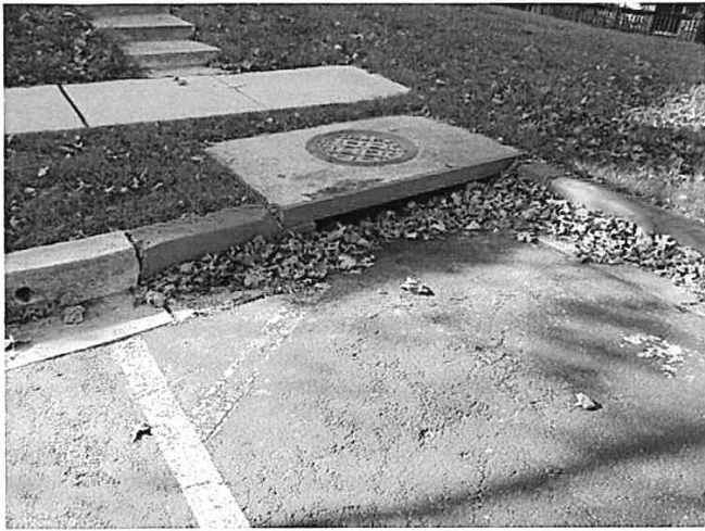
Typical catch basin
