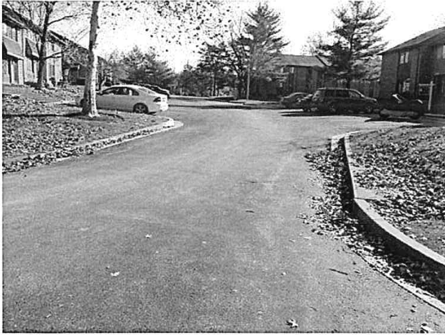
Chipwood Court pavement
