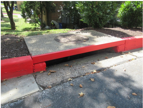
Catch basin overview
