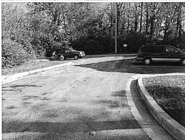
2005 parking lot pavement
