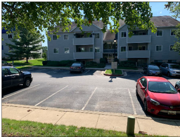
Photo 3: Sidewalk and asphalt conditions near buildings 2211 and 2212.
