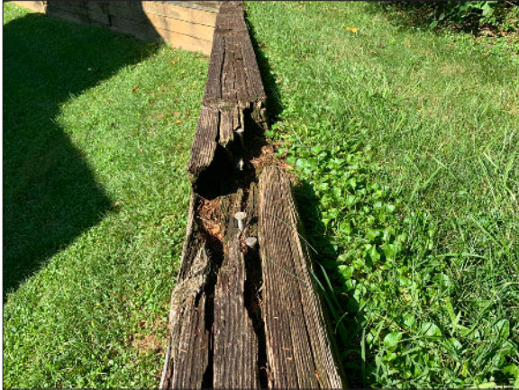
Photo 17: General conditions on the retaining wall in the rear of building 2212.
