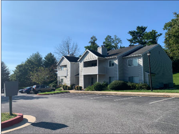
Photo 1: Building 2218 and general asphalt conditions.
