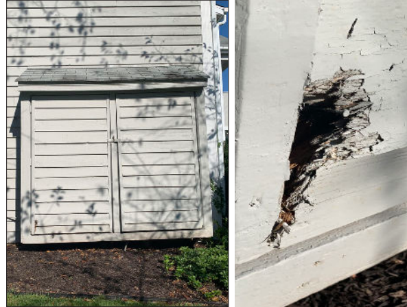
Photo 12: Utility room located on the southern side of building 2218. The damaged area highlighted is on the lower left corner of the doors.
