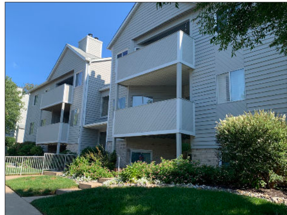
Photo 8: Typical example of the exterior of a three story building.
