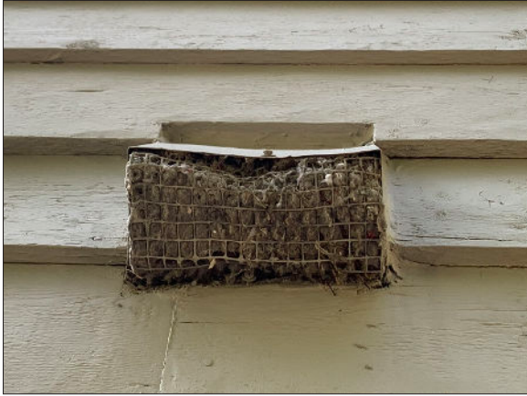
Photo 13: Example of an exterior vent which should be cleaned as part of regular annual maintenance.
