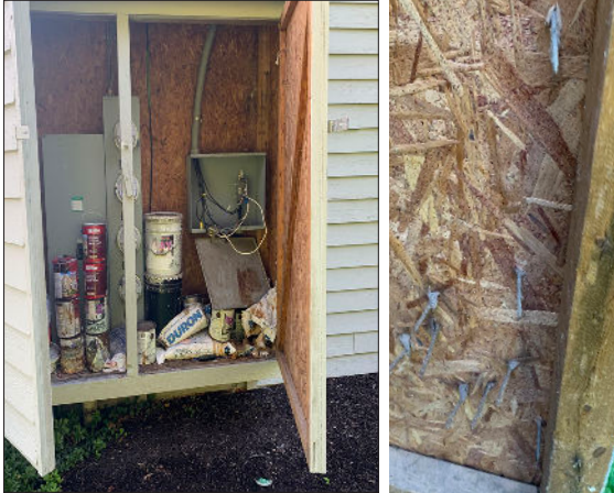
Photo 11: Utility room located on the northern side of building 2218. Note the nails on the inside of the utility room doors.
