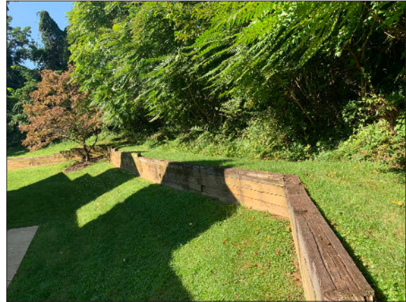
Photo 18: General conditions on the retaining wall in the rear of building 2212.
