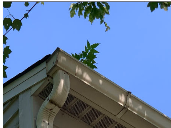
Photo 20: The gutters on building 2212.
