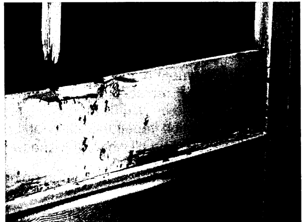
Wood trim deterioration at building 10
