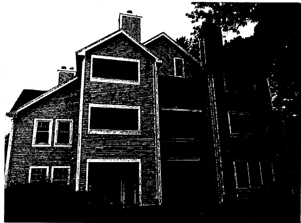
Three-story building overview
