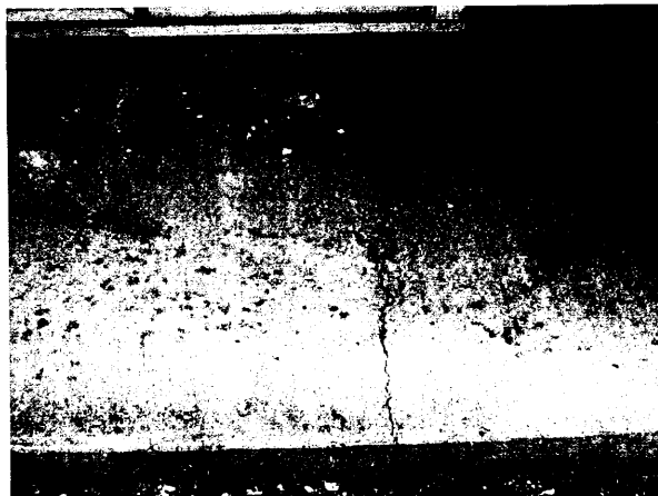
Concrete patio minor crack
