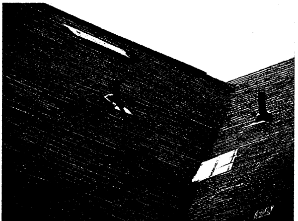
Missing and damaged shingles at building 4
