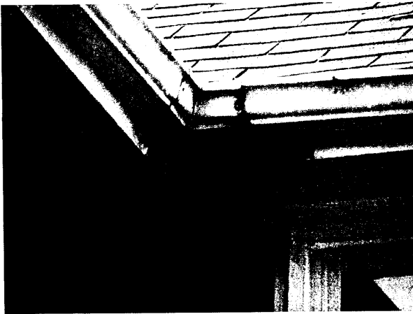
Evidence of gutter leaks at building 4
