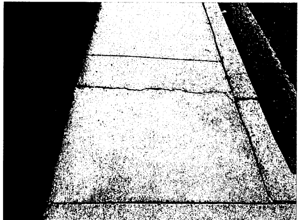
Concrete sidewalk cracks
