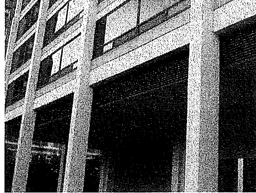
Concrete wall and columns
