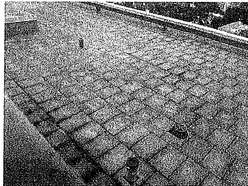
Inverted roof overview – Note: paver system
