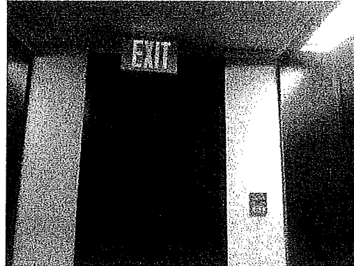
Life safety system devices
