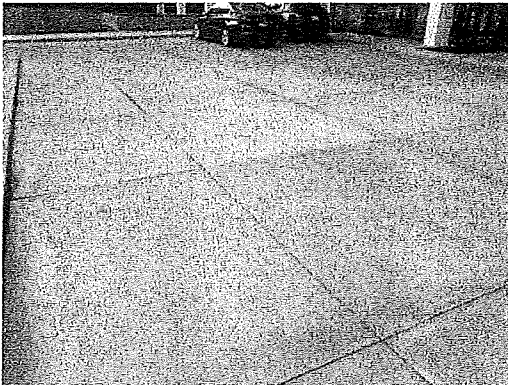
Concrete driveway at front
