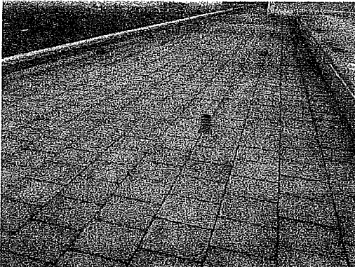
Inverted roof overview – Note: paver system
