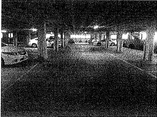
Concrete garage overview
