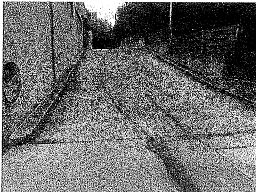
Concrete driveway at rear
