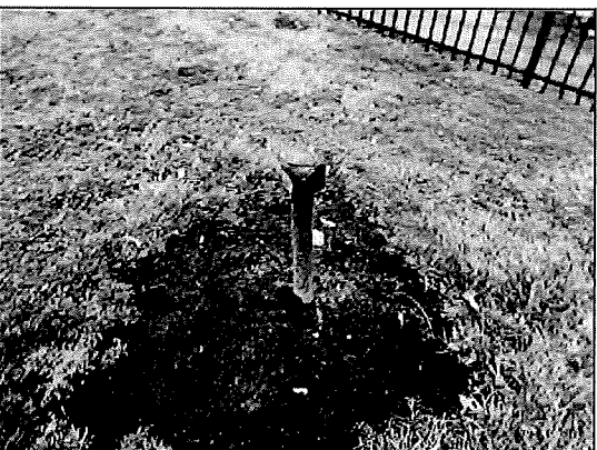
Photo #41. Improperly abandoned BBQ facilities near the swimming pool.
