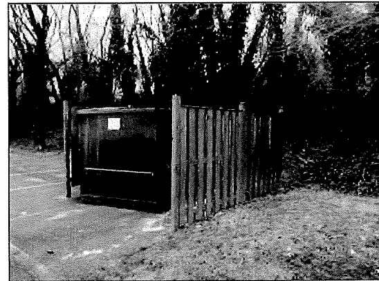
Photo #36. Partial replacement of trash corral fencing.
