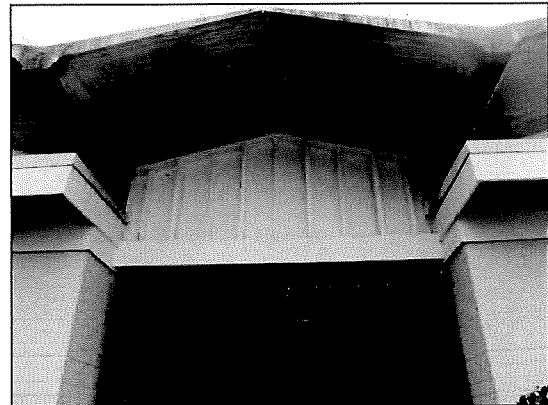
Photo #34. Detail view of the entrance to the Pool Building (PB).
