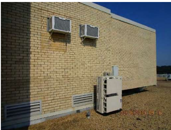
Photo 46: Elevator machine room heat pump condensing unit on roof and thru-wall air-conditioners (no longer used on Building 6631)
