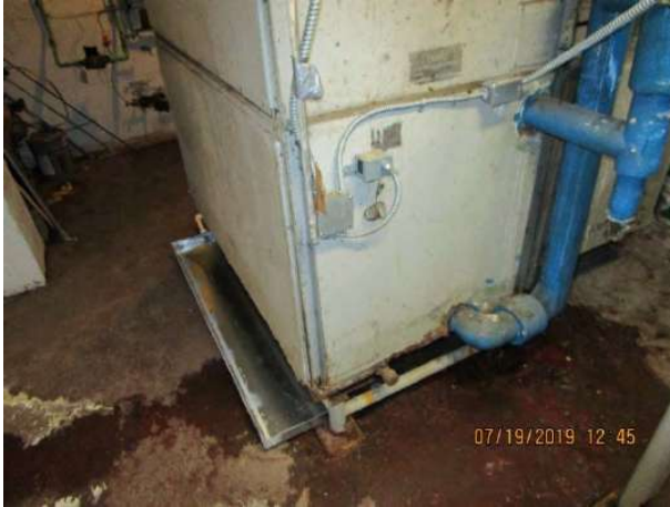
Photo 42: Corridor air handler in mechanical room in poor condition (Building 6631)
