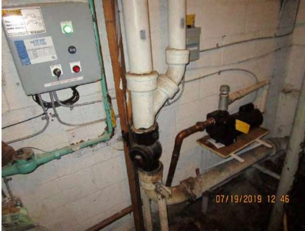
Photo 54: Elevator sump pump system (Building 6631)
