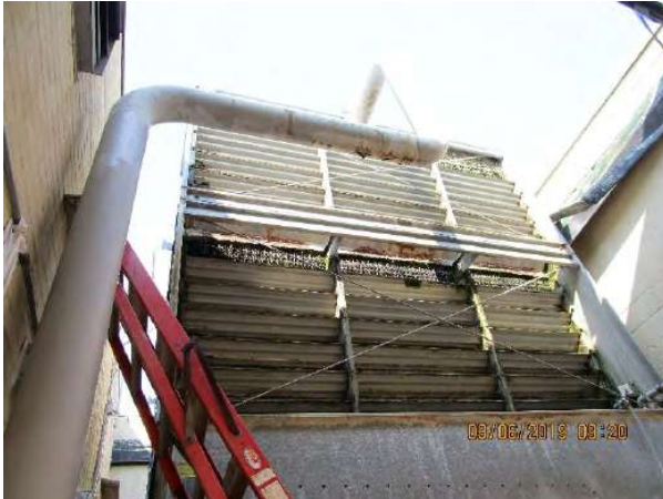
Photo 45: Cooling tower view of drift eliminators (Building 6631)
