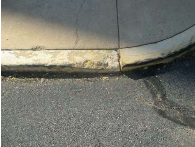
Photo 4: Spalled concrete curb and deteriorated paint
