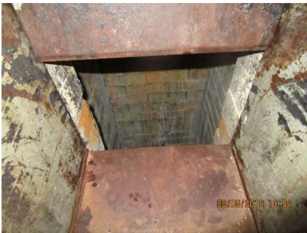
Photo 56: Typical trash chute interior
