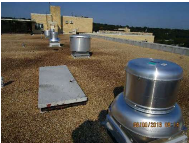
Photo 44: Roof exhaust ventilation fans viewed from eastern building edge (Building 6631)
