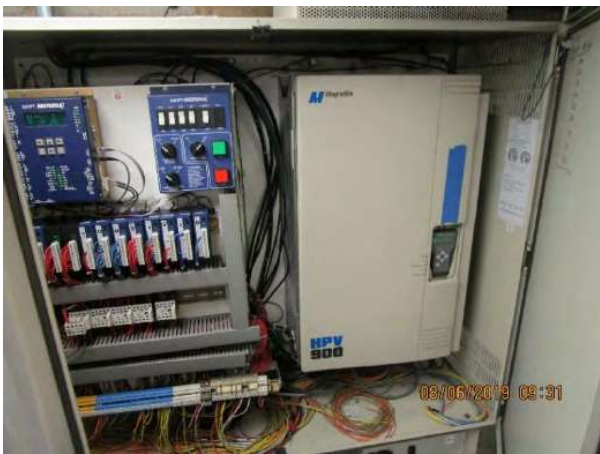
Photo 68: Elevator control panel installed by Elevator Control Equipment in 2012 (Building 6631)
