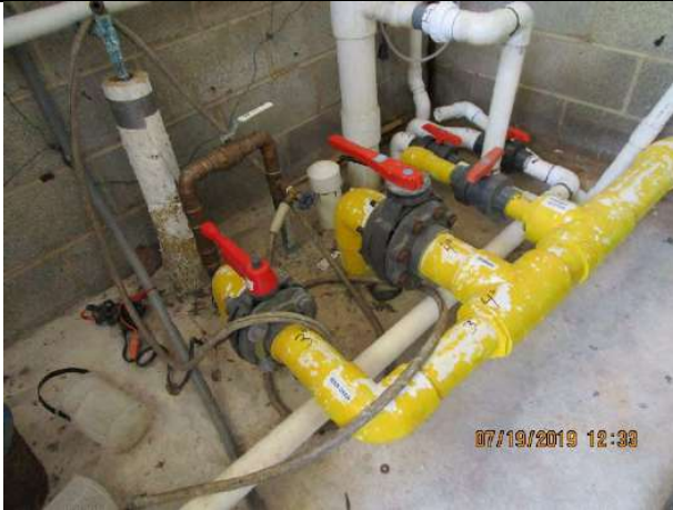
Photo 23: Pool water flow and isolation valves and piping distribution
