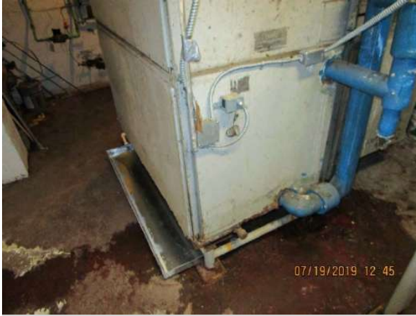
Photo 42: Corridor air handler in mechanical room in poor condition (Building 6631)
