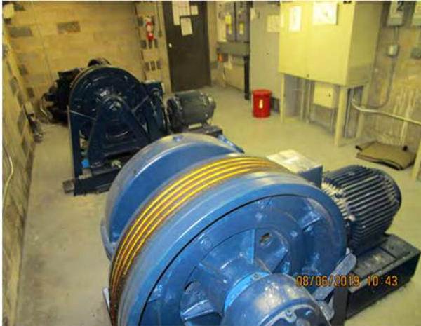
Photo 66: Typical elevator machine room and elevator motors with cabling
