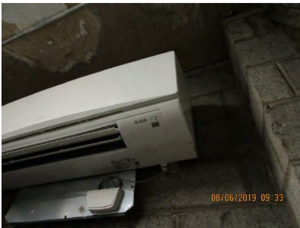
Photo 67: Elevator machine room cooled by ductless split system (Building 6631)
