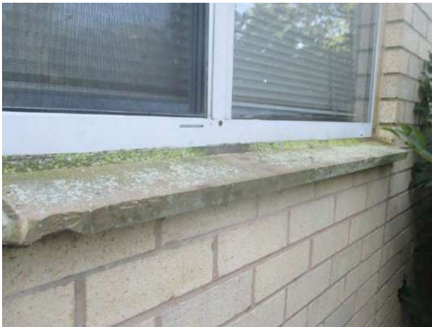
Photo 33: Typical window and concrete window sill
