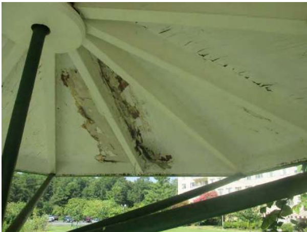
Photo 15: Deteriorated wood umbrella at outdoor seating area
