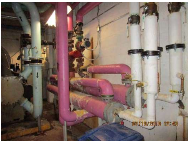
Photo 53: Tube in shell heat exchangers for domestic hot water (Building 6631)
