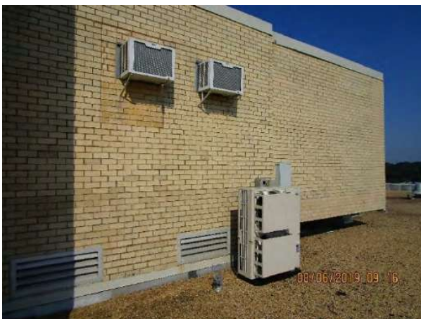
Photo 46: Elevator machine room heat pump condensing unit on roof and thru-wall air-conditioners (no longer used on Building 6631)
