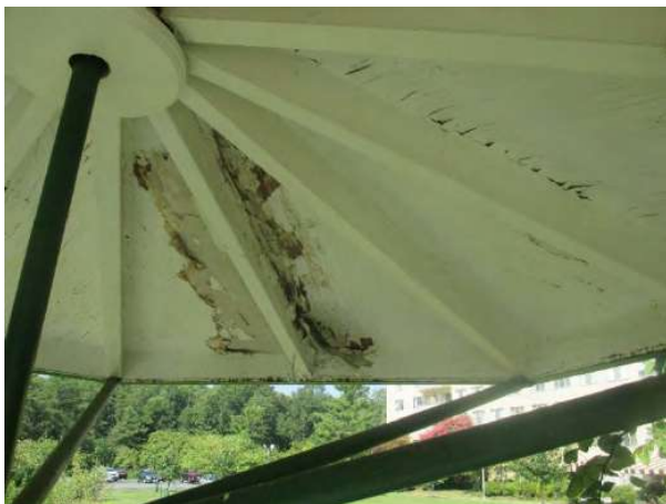
Photo 15: Deteriorated wood umbrella at outdoor seating area
