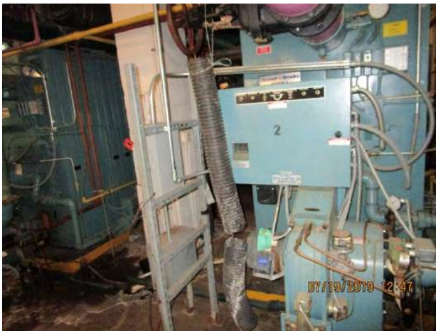
Photo 43: Heating hydronic boilers – dual fuel (Building 6631)
