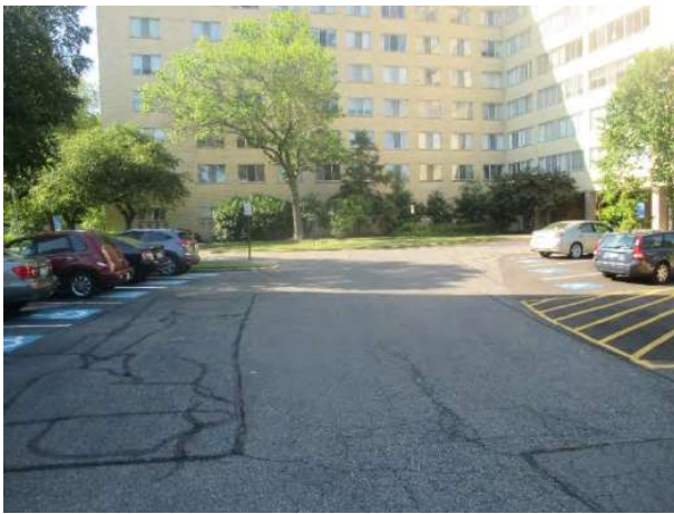
Photo 2: Alligator cracks and previously repaired parking stalls at Building 6631
