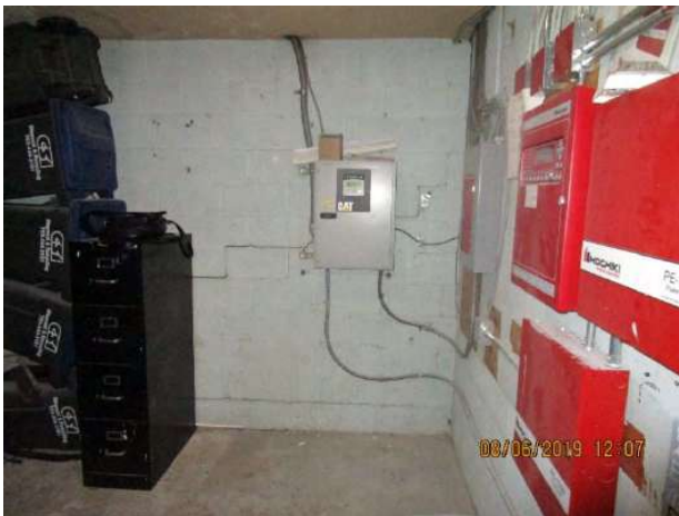
Photo 55: Building 6631 Hochiki PE-10SN fire alarm installed in 2014 (typical of the three building systems)
