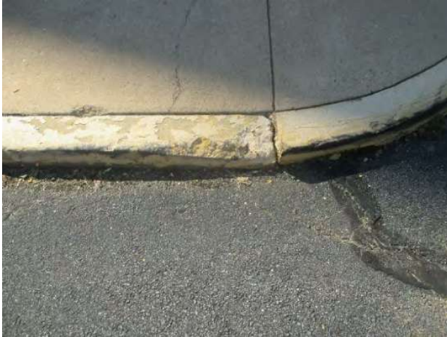
Photo 4: Spalled concrete curb and deteriorated paint
