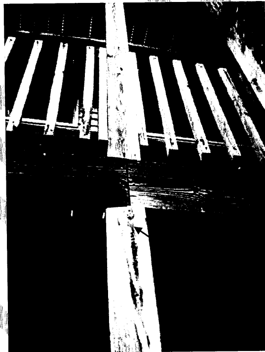
Photograph #4: Warped Walkway Post at Rim Joist Connection
